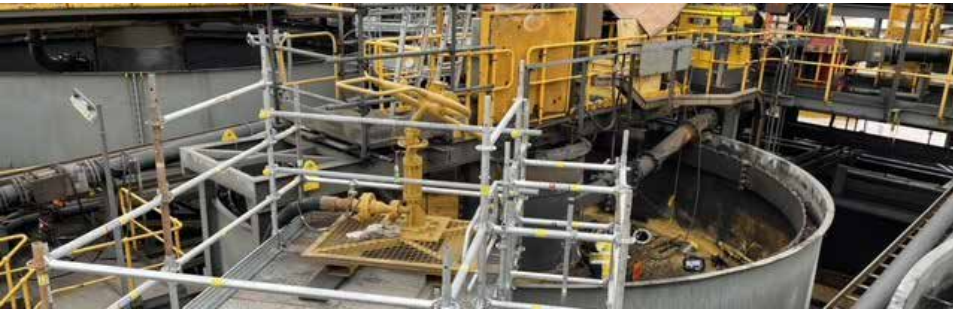
Tank and Thickner Cleaning
